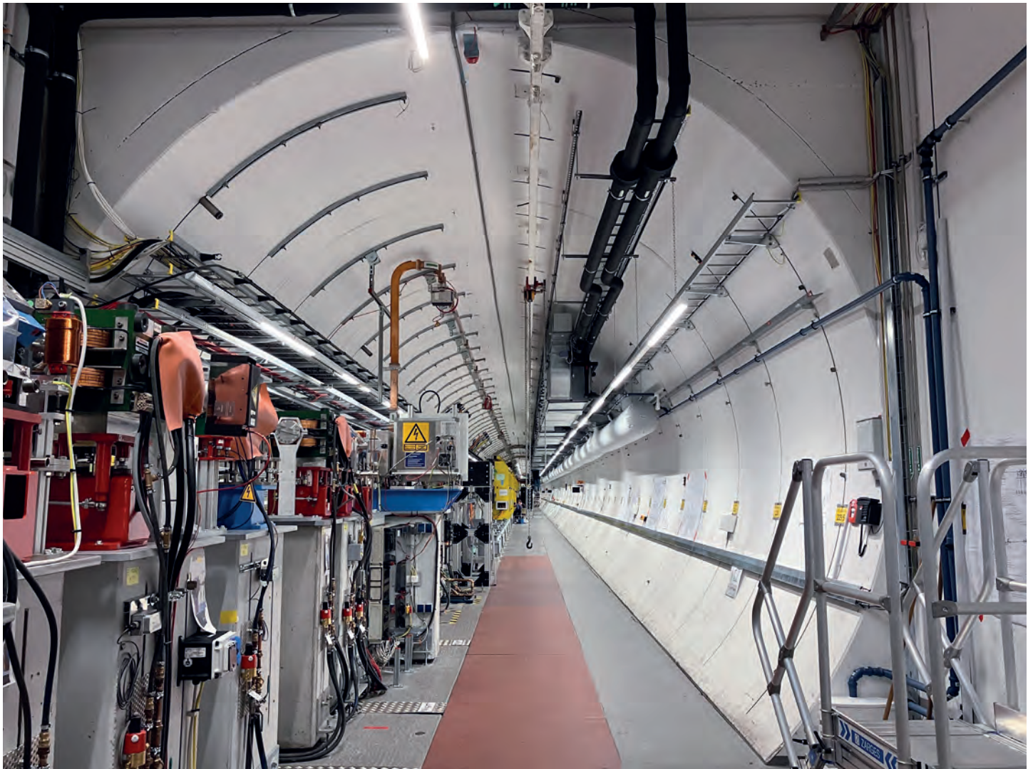
Figure 2 View into the full FLASH1 tunnel a few days before the restart on 4 August 2025. Over a length of about 120 m, the new electron beamline, undulators, laser and photon beamlines and all the related infrastructure, such as AC, cooling water, electricity and IT-networks were installed. (Credit: DESY)
