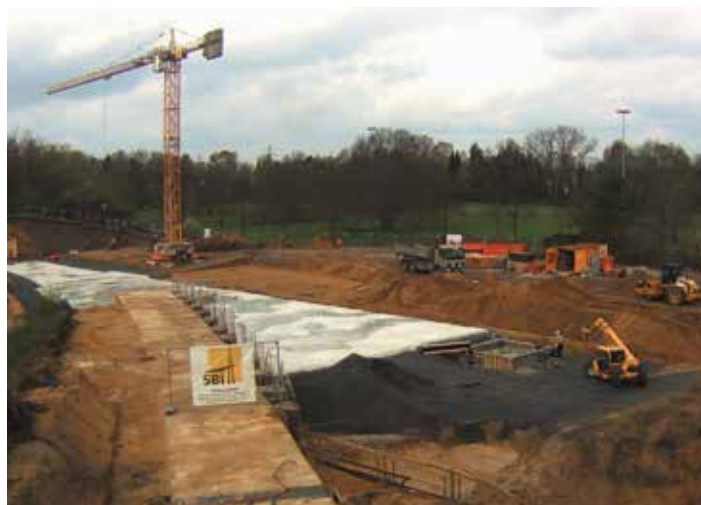
The civil construction work for the PETRA III extension hall North started with removing the soil that covers the storage ring tunnel in that area.
