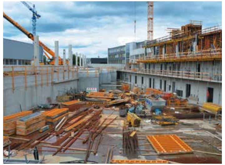
Figure 8 Civil engineering of hall east (August 2014).
