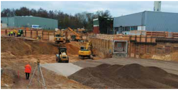
Figure 6 Digging at the site of hall east. The remaining tunnel is seen on the right (March 2014).
