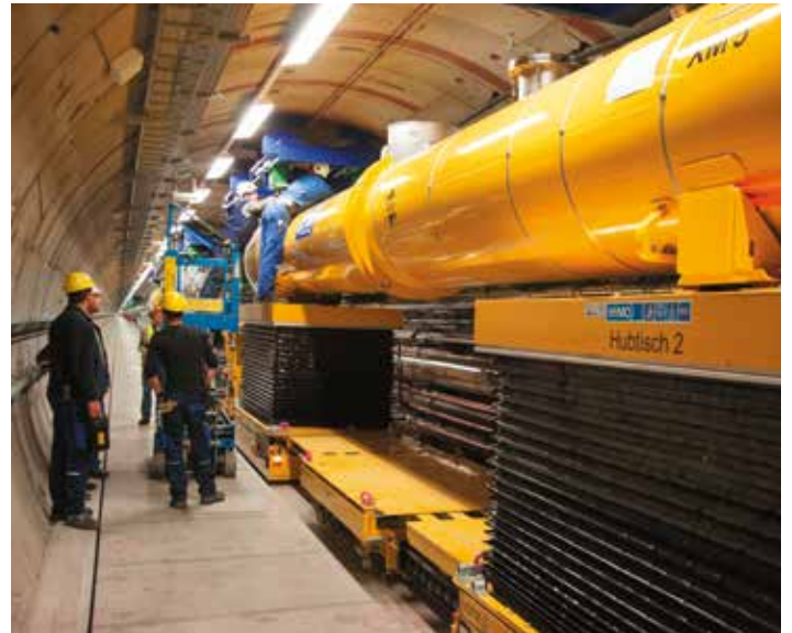
Installation of one of the first accelerator modules in the tunnel of the European XFEL by workers of the DESY-led Accelerator Consortium.
