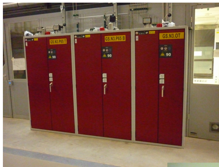
Gas cabinets for toxic, inflammable and oxidising gases
