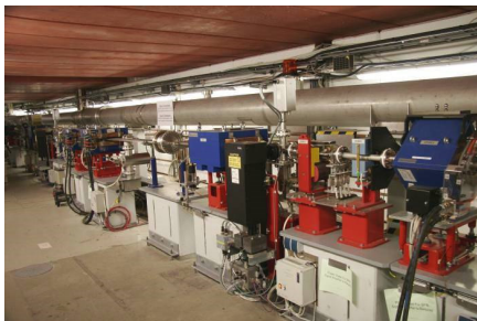
Bunch Compressors (Magnetic Chicane, Current increase 50A → 1000 A)
